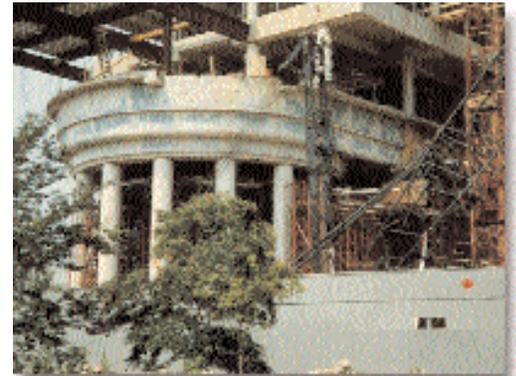
*Figure 1: Greening occurred in concrete made with slag cement after forms were removed on the Canadian Chancery in Washington, D.C.*
