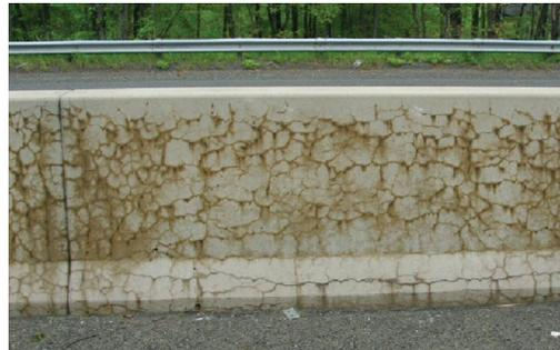
Fig. 1: ASR causes expansion and cracking of concrete structures and pavements
