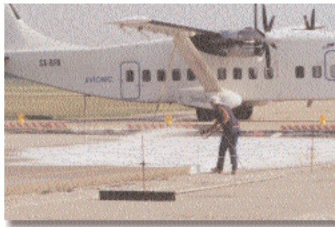
Figure 3: As with all concrete, proper curing practices are essential.
