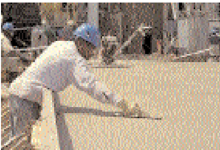
Figure 2: Finishing is usually enhanced with slag cement
