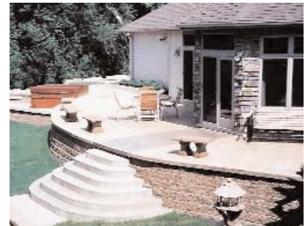
Completed exterior of a home with insulating concrete forms, in Wisconsin.
