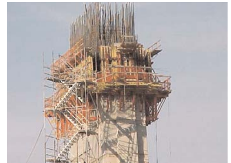
Reliant Stadium (NFL) in Houston, which opened in 2002, used a portland-slag cement-fly ash mixture to achieve both high strength and low heat in its four massive "super columns," supporting the retractable roof.
