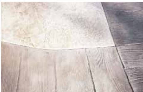
Decorative residential concrete with 25 percent slag cement: Interior acid stained concrete (top) and exterior stamped and colored concrete (bottom)
