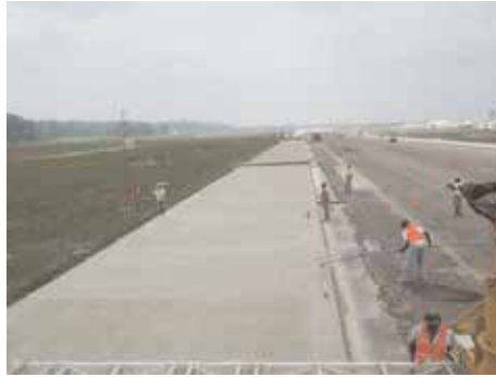
Airport paving at Spirit of St. Louis Airport in Chesterfield, MO, placed with blended cement (Type 1 (SM)) and Class C Fly Ash added separately.
