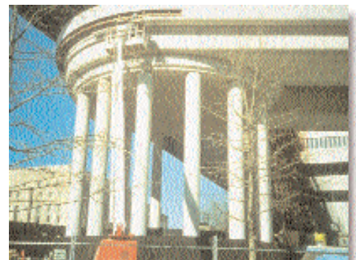
Figure 2: Exposure to sunlight and air allowed the concrete surface at the Canadian Chancery to oxidize and lighten.
