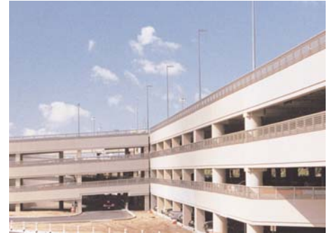
Figure 1: Slag cement not only reduces energy, emissions and virgin material requirements in concrete, it also lightens the concrete, so exposed concrete surfaces reflect more light and help reduce the urban heat island effect.
